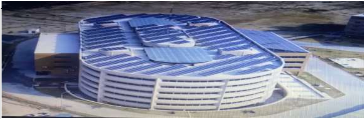
Installed Solar System at AUAACK
